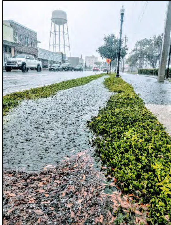
Figure 2-2. Photo of a raingarden capturing runoff and road debris in downtown Winter Haven.
