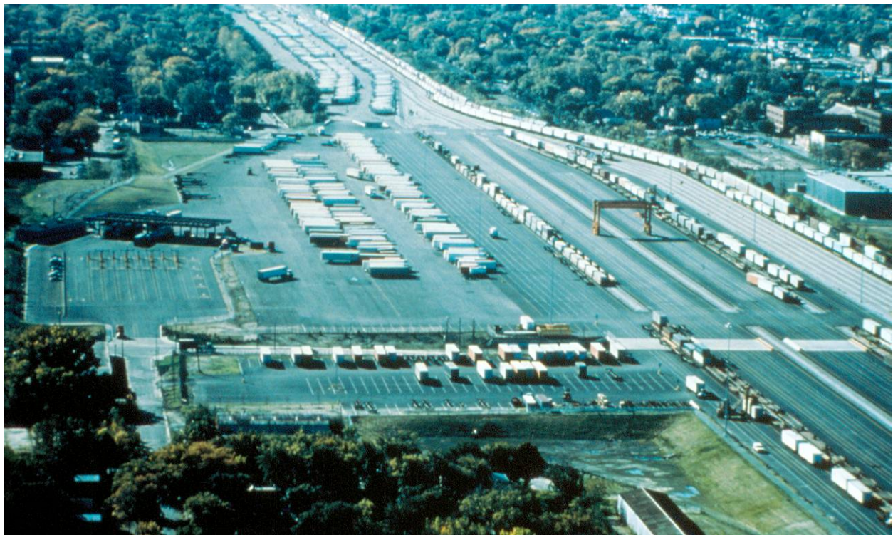
CSX Intermodal terminal at 59th Street in Chicago
