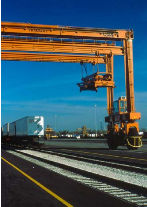
CSX Intermodal Terminal at 59 th Street, Chicago
