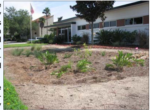
A rain garden under construction at the East City Hall Annex.
